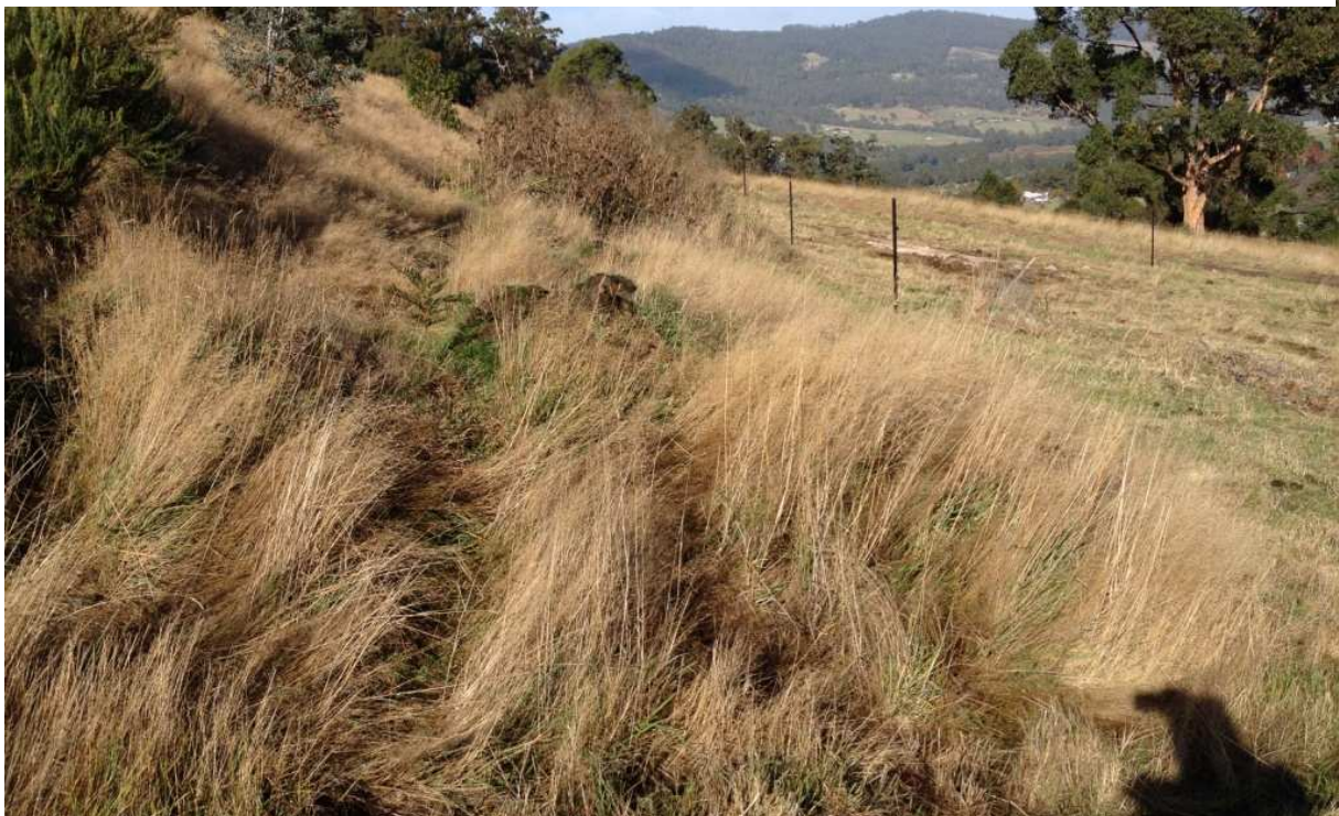
Plate 2 (below). Topsoil from the house excavation stockpiled at the base of the embankment is suitable for a non-conventional bed, provided its grass cover is destroyed before emplacement.
