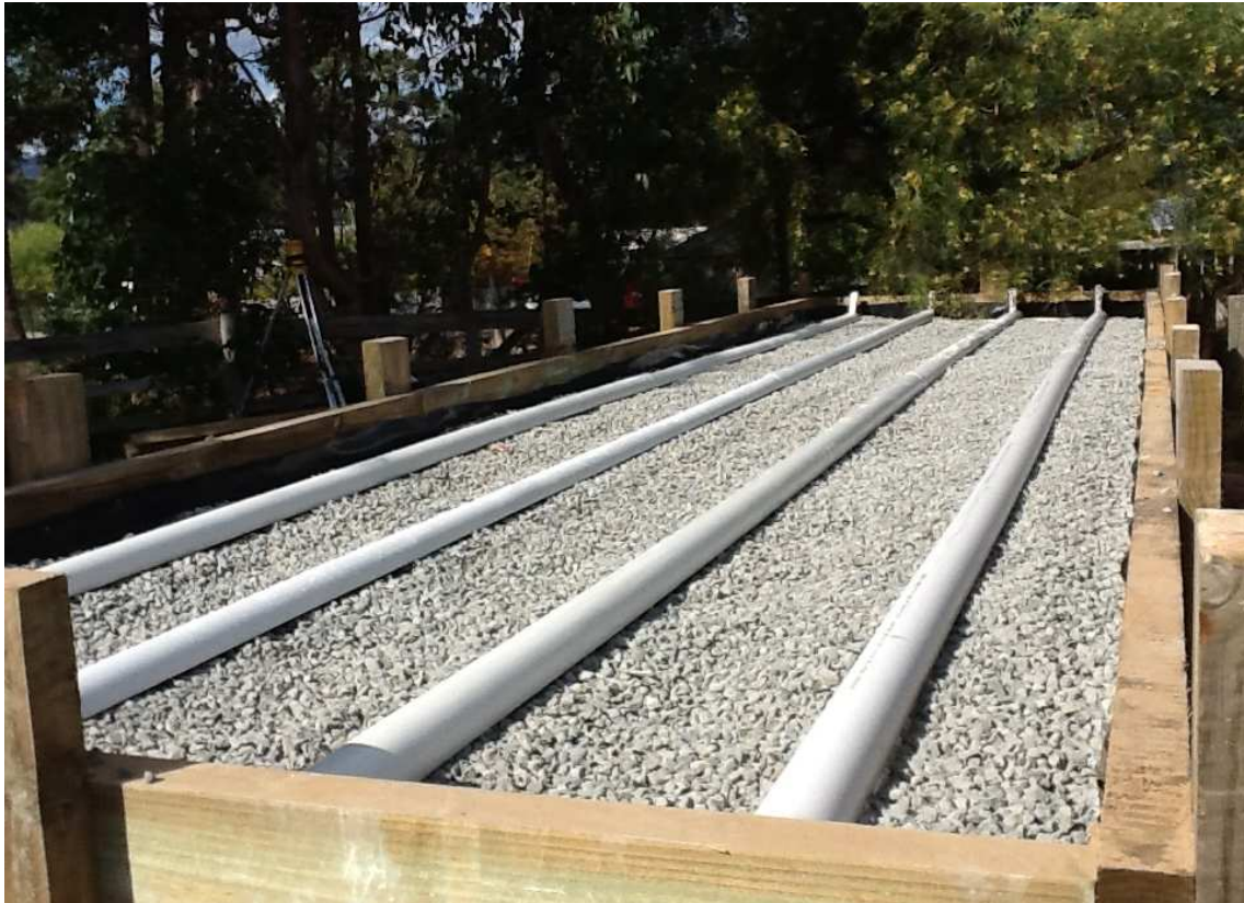
Plate 11 (above). Half-pipe 100mm Class 9 UPVC over 40mm distribution grid
