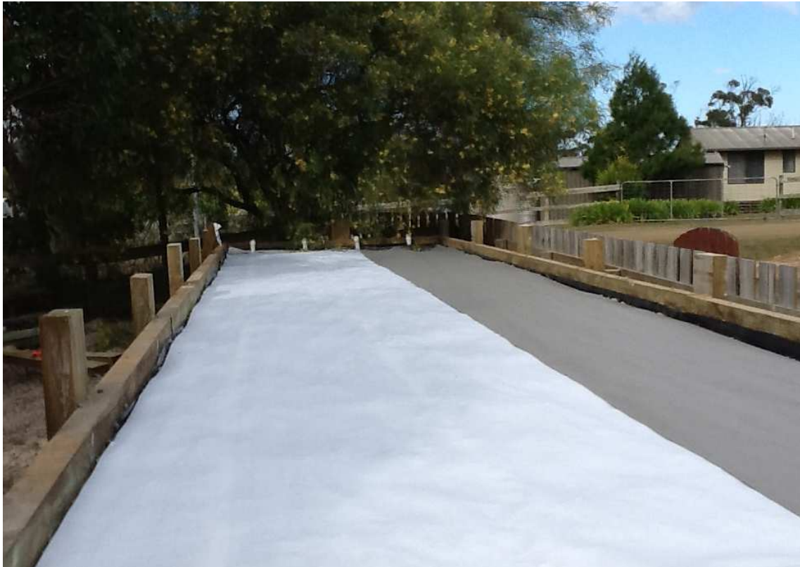
Plate 13 (above). Geofabric in place over aggregate
