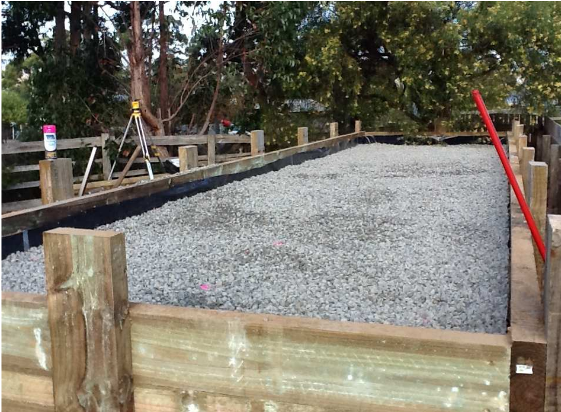
Plate 7 (above). Screened aggregate complete
