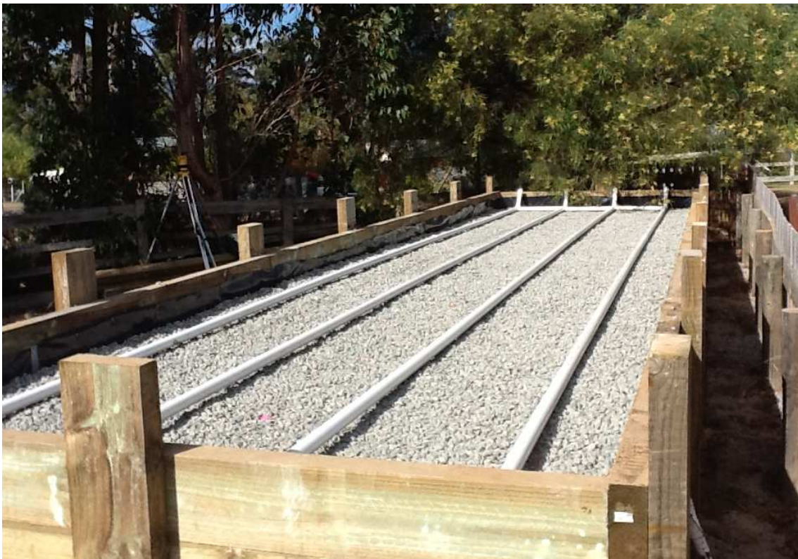
Plate 8 (below). Grid of 40mm Class 9 UPVC pipework in place, with raised inspection openings at far end.
