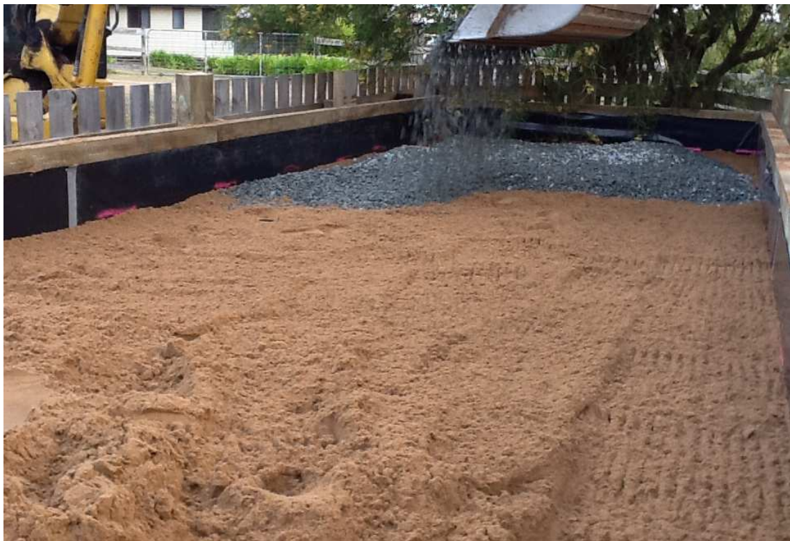
Plate 6 (below). Filter sand complete. Screened aggregate being placed.
