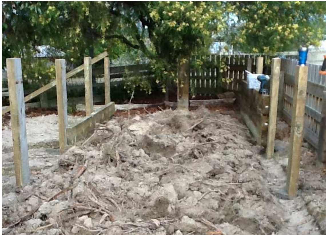
Plate 3 (above). Ripping completed.
