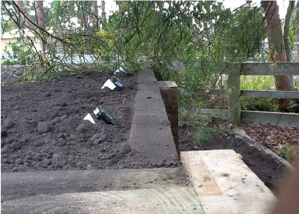
Plate 15 (above). Inspection openings
