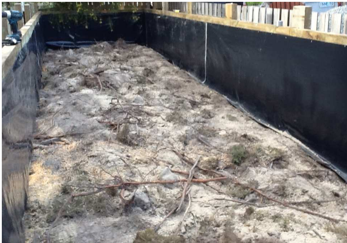
Plate 4 (below). Fencing and plastic liner completed. Note vertical seal on liner.
