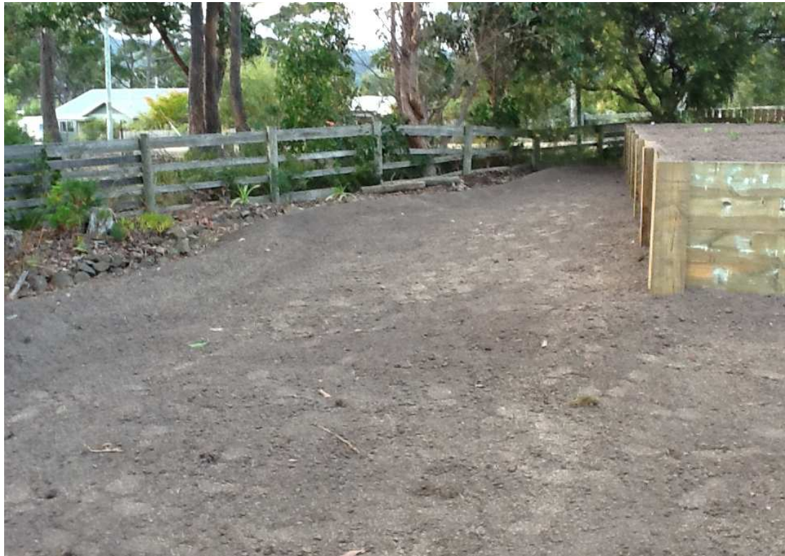
Plates 17 (above) and 18 (below). Apron of Category 1, 2, 3, or 4 placed on downslope and sides of basic module. Shrubs and grass to be planted.
