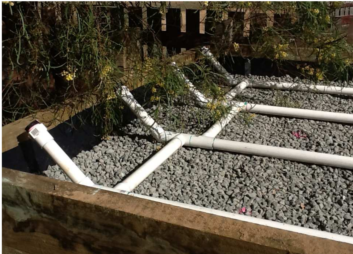
Plate 9 (above). Inspection openings.
