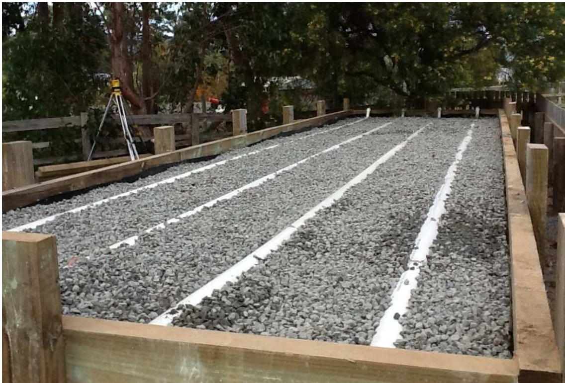
Plate 12 (below). Pipework covered with aggregate. Horizontal galvanised 10mm rods tie each second pair of opposite posts together.
