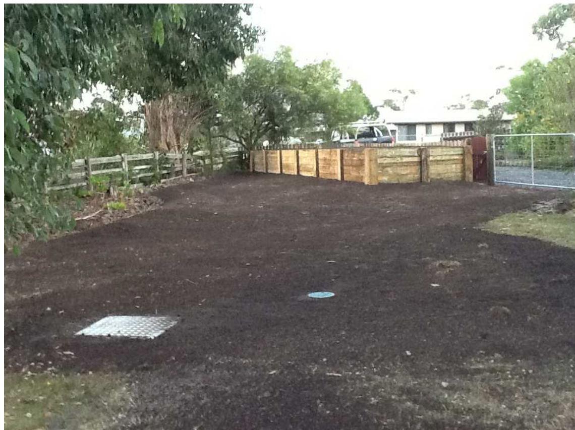
Plates 17 (above) and 18 (below). Apron of Category 1, 2, 3, or 4 placed on downslope and sides of basic module. Shrubs and grass to be planted.
