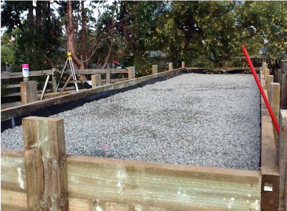
Plate 7 (above). Screened aggregate complete
