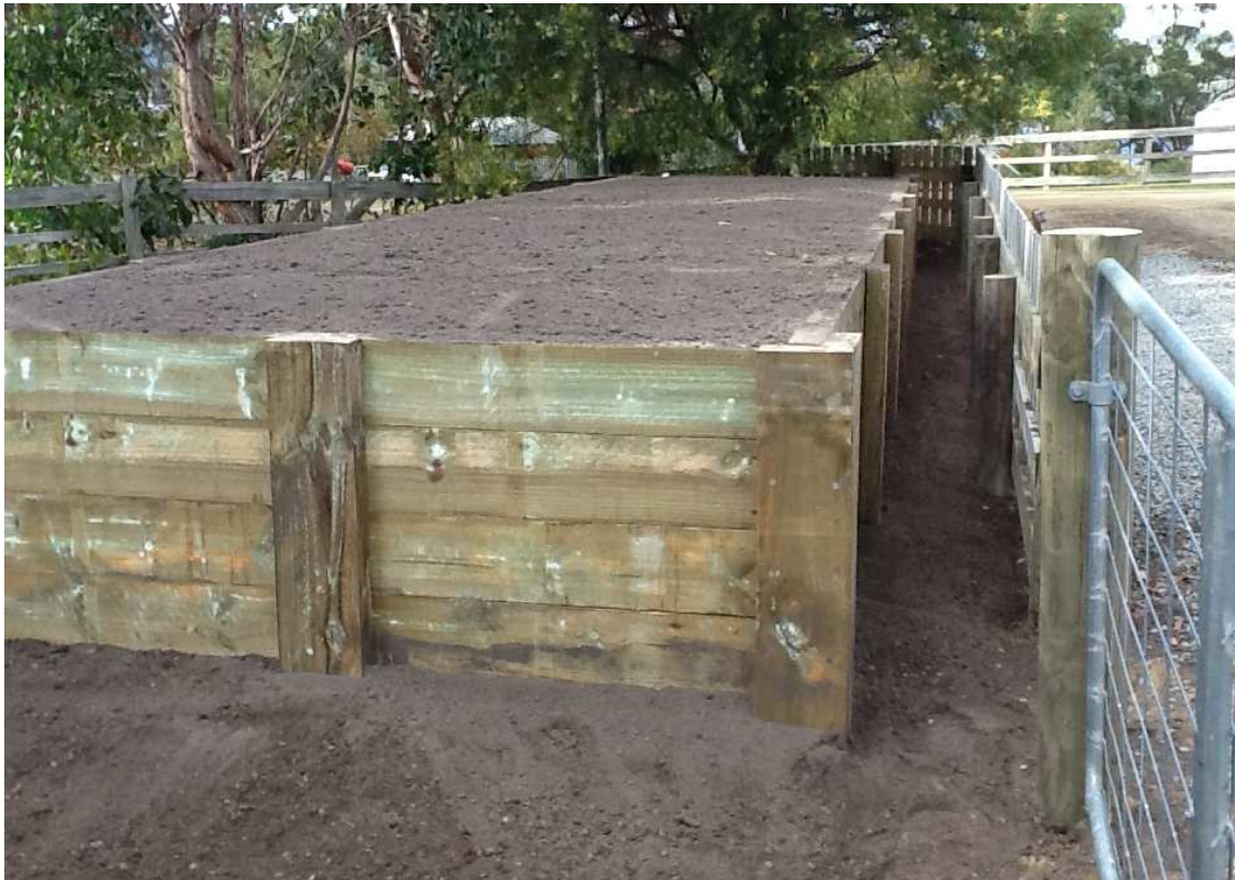
Plate 14 (below). Final loam layer in place prior to planting.
