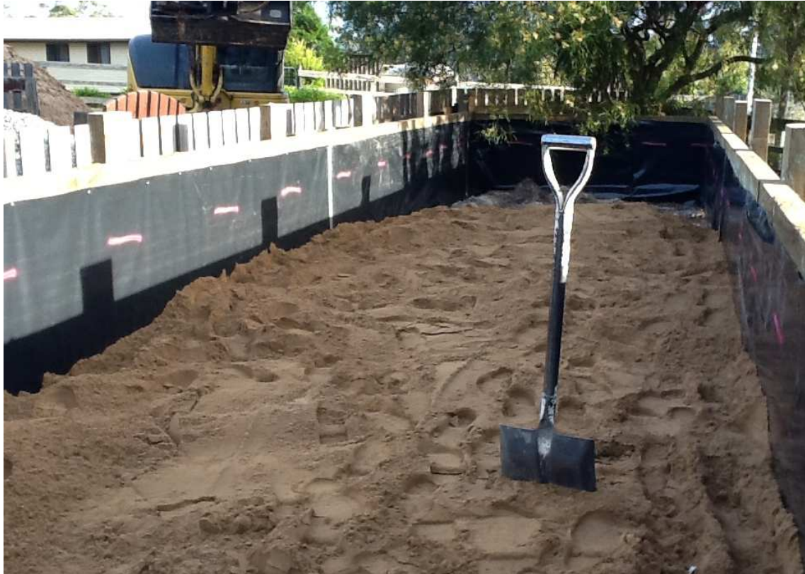
Plate 5 (above). Placement of filter sand. Lay in nom. 100mm layers; walk over to slightly compact, especially against plastic around edges.
