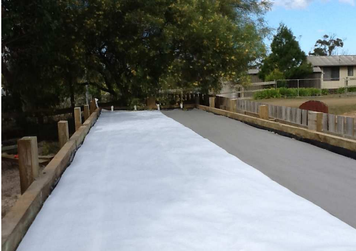
Plate 13 (above). Geofabric in place over aggregate
