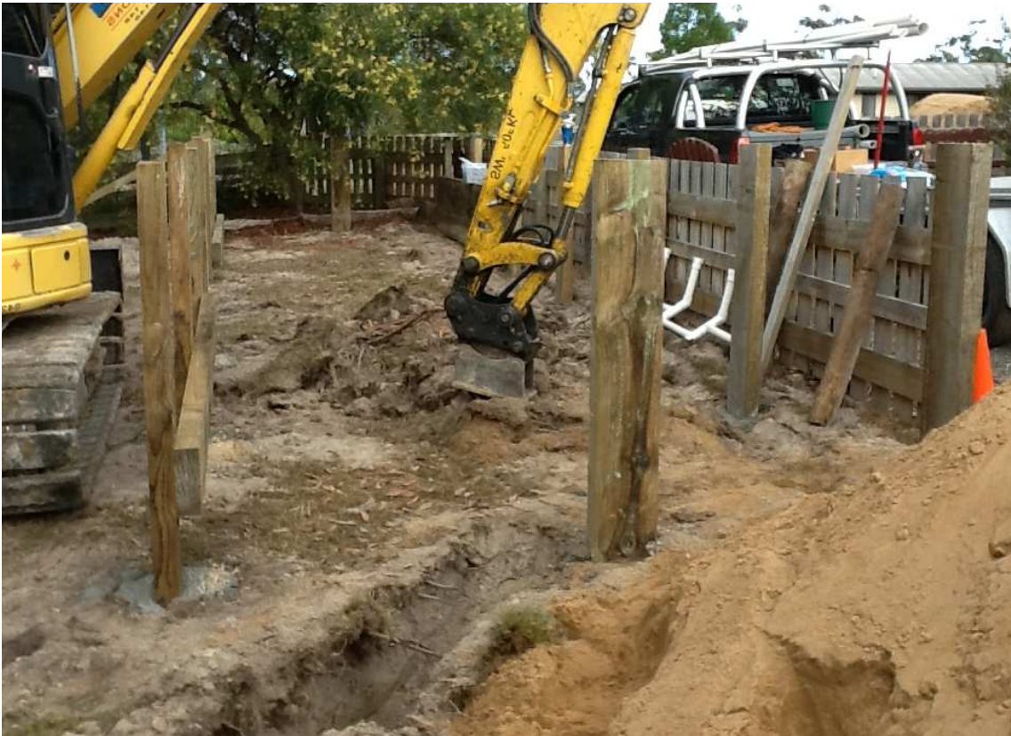
Plate 2 (below). Ripping soil over the base of the basic module. Filter sand in right foreground.
