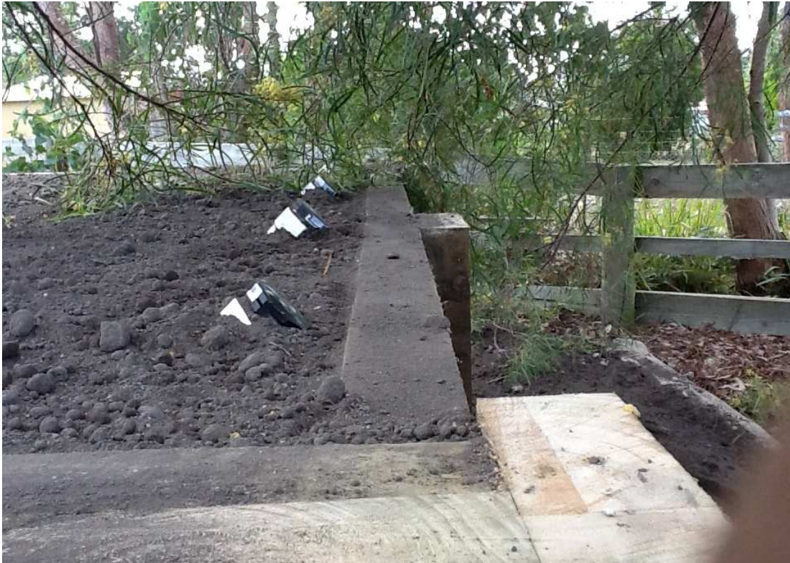
Plate 15 (above). Inspection openings
