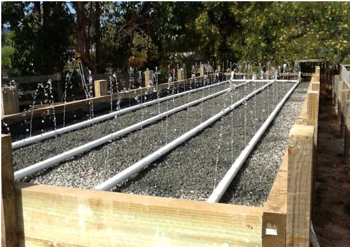
Plate 10 (below). Perforated pipework under test with clean water.
