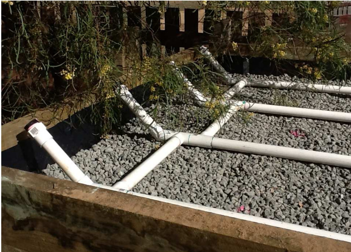
Plate 9 (above). Inspection openings.
