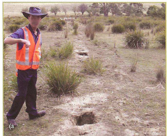
Figure 5. Piping failure or tunnel erosion in a dam constructed from soils derived from Permian mudstone. This dam is known to have failed on first filling. The image was taken from the dam floor.
